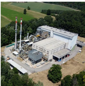
- IT_0013 - CREMONA INCINERATION PLANT - AEM CREMONA SPA - 76,569 tonnes. 6.1MWe, 35.6MWt
