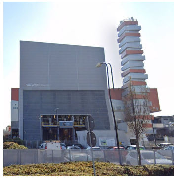
- IT_0034 - PADOVA INCINERATION PLANT - HERA AMBIENTE - 169,251 tonnes. 18.1MWe, 79.8MWt
