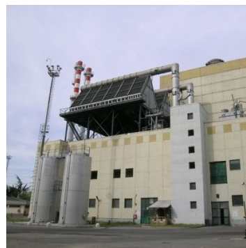
- IT_0008 - BUSTO ARSIZIO INCINERATION PLANT - ACCAM SPA - 80,263 tonnes. 11MWe, 61MWt
