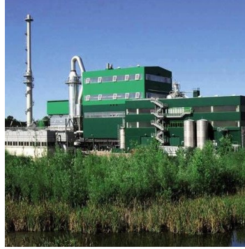
- IT_0012 - CORTEOLONA INCINERATION PLANT - A2A AMBIENTE SPA - 69,413 tonnes. 8.1MWe, 34MWt
