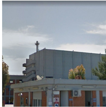
- IT_0050 - STATTE INCINERATION PLANT - AMIU SPA - 66,600 tonnes. 3.5MW e
