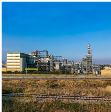
- IT_0027 - MELFI INCINERATION PLANT - FENICE SPA - 36,151 tonnes. 7.3MWe, 50.1MWt
