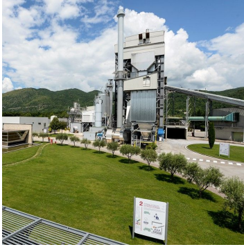
- IT_0041 - POZZILLI INCINERATION PLANT - ENERONUT SPA - 85,039 tonnes. 13.2MWe, 47MWt
