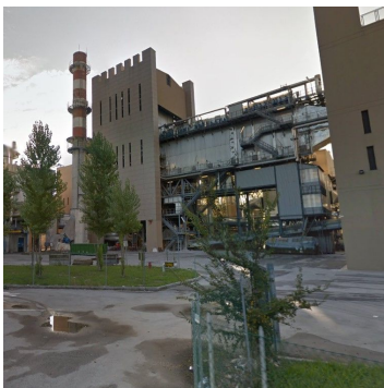
- IT_0011 - RIMINI (CORIANO) INCINERATION PLANT - HERA SPA - 147,663 tonnes. 13MWe, 46.5MWt
