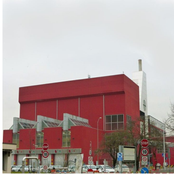
- IT_0019 - FORLÌ INCINERATION PLANT - HERA SPA - 119,993 tonnes. 10.6MWe, 46.5MWt
