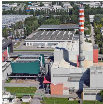
- IT_0016 - FERRARA - CASSANA INCINERATION PLANT - HERA SPA - 129,912 tonnes. 13MWe, 55.8MWt
