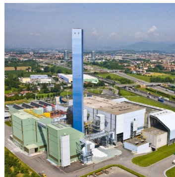
- IT_0006 - BRESCIA INCINERATION PLANT - A2A AMBIENTE - 721,167 tonnes. 117MWe, 305MWt
