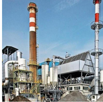
- IT_0048 - SCHIO INCINERATION PLANT - ALTO VICENTINO AMBIENTE SRL - 86,055 tonnes. 6.7MW e , 39.3MWt
