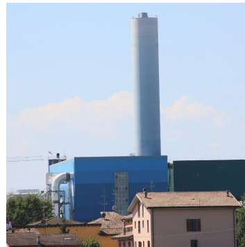
- IT_0030 - MODENA INCINERATION PLANT - HERA SPA - 211,326 tonnes. 24.8MWe, 78MWt
