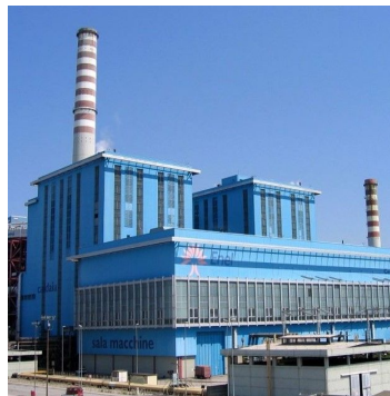
- IT_0020 - FUSINA INCINERATION PLANT - VERITAS - 80,000 tonnes. 16MWe, 47.8MWt
