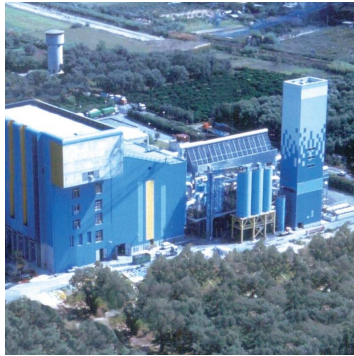
- IT_0021 - GIOIA TAURO INCINERATION PLANT - VEOLIA SERVIZI AMBIENTALI SPA - 39,965 tonnes. 17.3MWe, 60MWt
