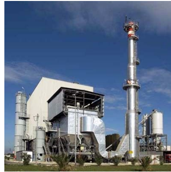
- IT_0026 - MASSAFRA INCINERATION PLANT - APPIA ENERGY - 60,524 tonnes. 12.3MWe, 49.5MWt
