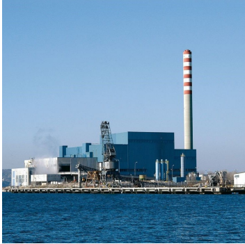
- IT_0055 - TRIESTE INCINERATION PLANT - ACEGAS APS - 154,511 tonnes. 17.5MW e , 67.3MWt
