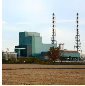
- IT_0036 - PARONA INCINERATION PLANT - LOMELLINA ENERGIA SRL PARONA - 230,194 tonnes. 44.8MWe, 147.8MWt
